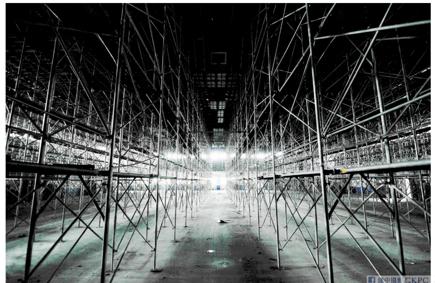
refurbishment of school stadium ▼
